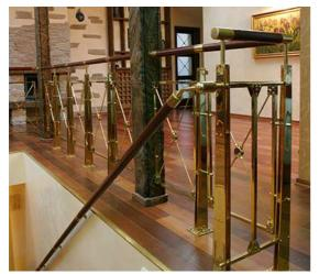
Stairs fencing made of polished brass. The key feature of this fencing is the rivet assembly. Elements of industrial style in the railing make it look like a complex and elegant product.
